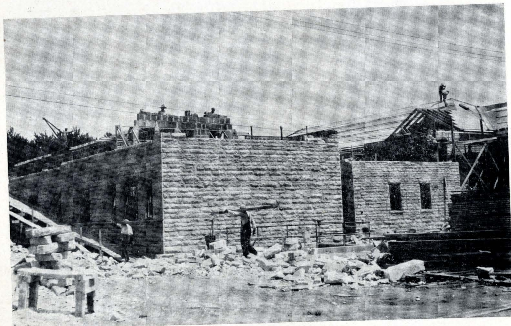
BUILDING CONSTRUCTION—HOME FIVE
