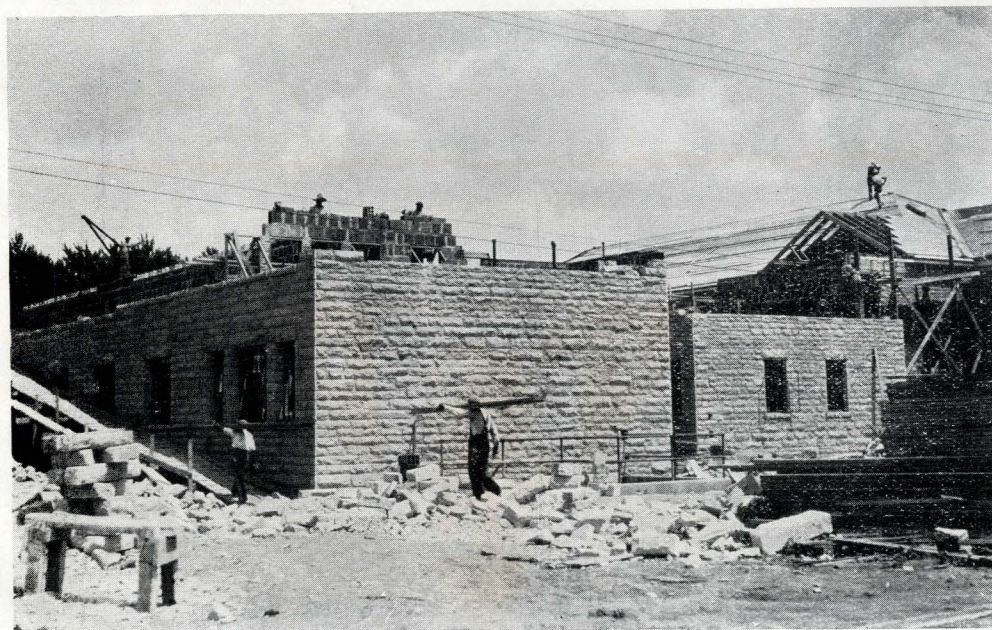
BUILDING CONSTRUCTION — HOME FIVE
