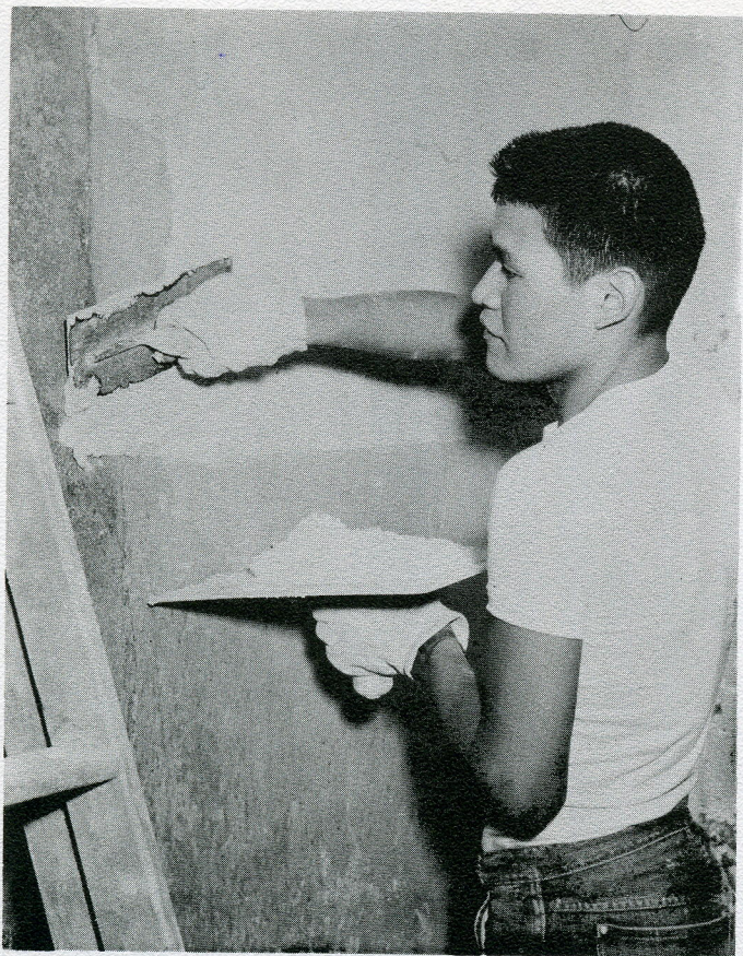
Ben Peters, student from the Masonry shop, plasters a campus building.
