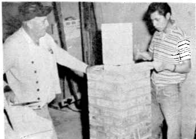
Instructor, Mr. Clifton Dee, watches Sandy Frye as he builds a six-brick flue.
