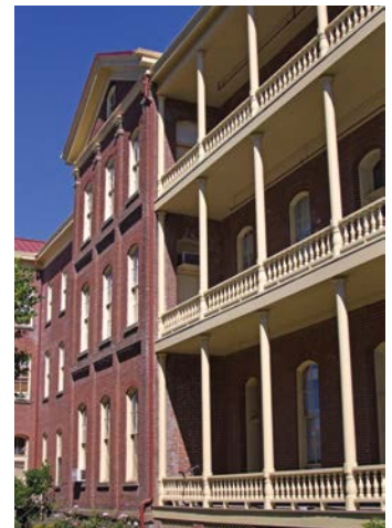
Figure 1: The installation of an exterior automatic fire sprinkler system for the historic multi-story porches allowed these important, character-defining features to be retained to meet life and fire-safety code requirements. Photo: Robert Holcomb
