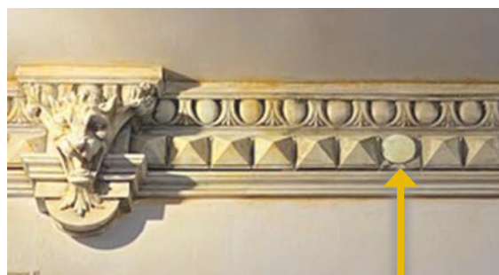
Figure 2: Sprinkler heads and other equipment can be selected and placed to have minimal visual intrusion with no impact on functionality, such as these fixed (left) or concealed (right, with arrow) sprinkler heads. Photos: Marilyn Kaplan
