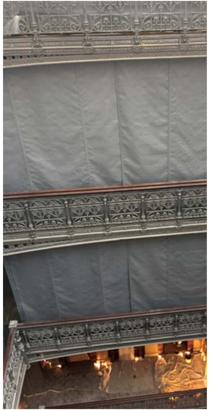
Figure 21. The photograph on the right illustrates partial deployment of vertical fire curtains activated as part of a fire alarm and detection system. In this installation, a combination of fixed glazing and smoke curtains to separate the open corridors from the multi-story atrium permitted the stunning historic atrium space to remain largely unaltered and the corridors to be included in the building's egress calculations in meeting code requirements. Photo: Higgins Quasebarth & Partners, LLC
