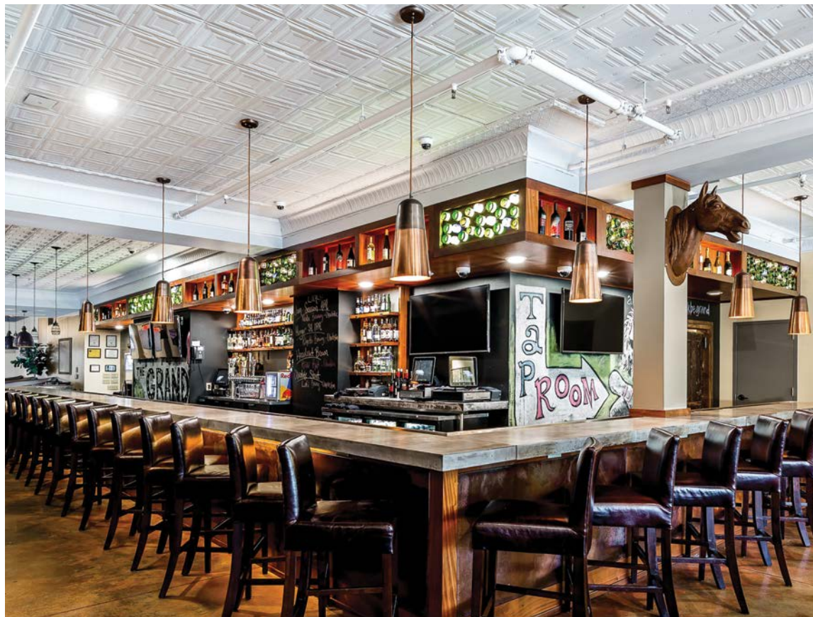
Figure 17. Metal ceilings commonly present code challenges when fire separation is required between different uses on the first and upper floors. Acceptable code solutions permitting retention may include the application of intumescent coatings, the addition of a sprinkler system, or the addition of fire-rated material above the ceiling, in which case the original metal ceilings can be salvaged and reinstalled or, if not possible, replaced with matching new ceiling tiles. Photo: Benton Henry
