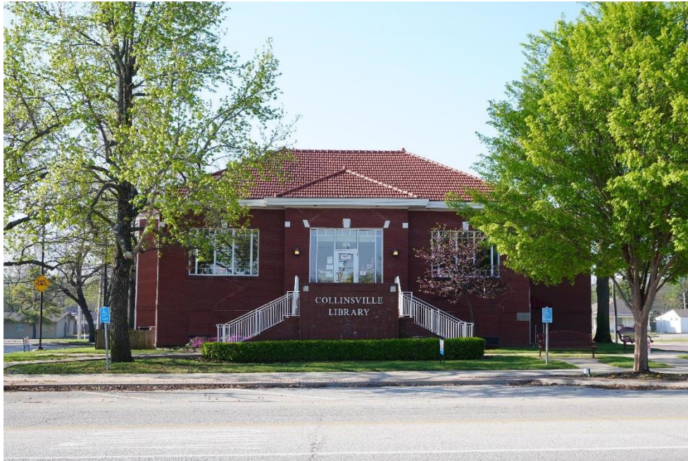
Figure 10: 1223 West Main Street
