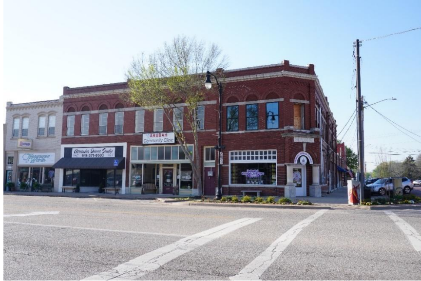
Figure 8: 1023 West Main Street
