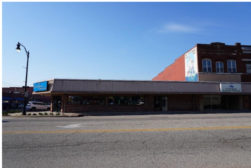
Figure 9: 1101 West Main Street
