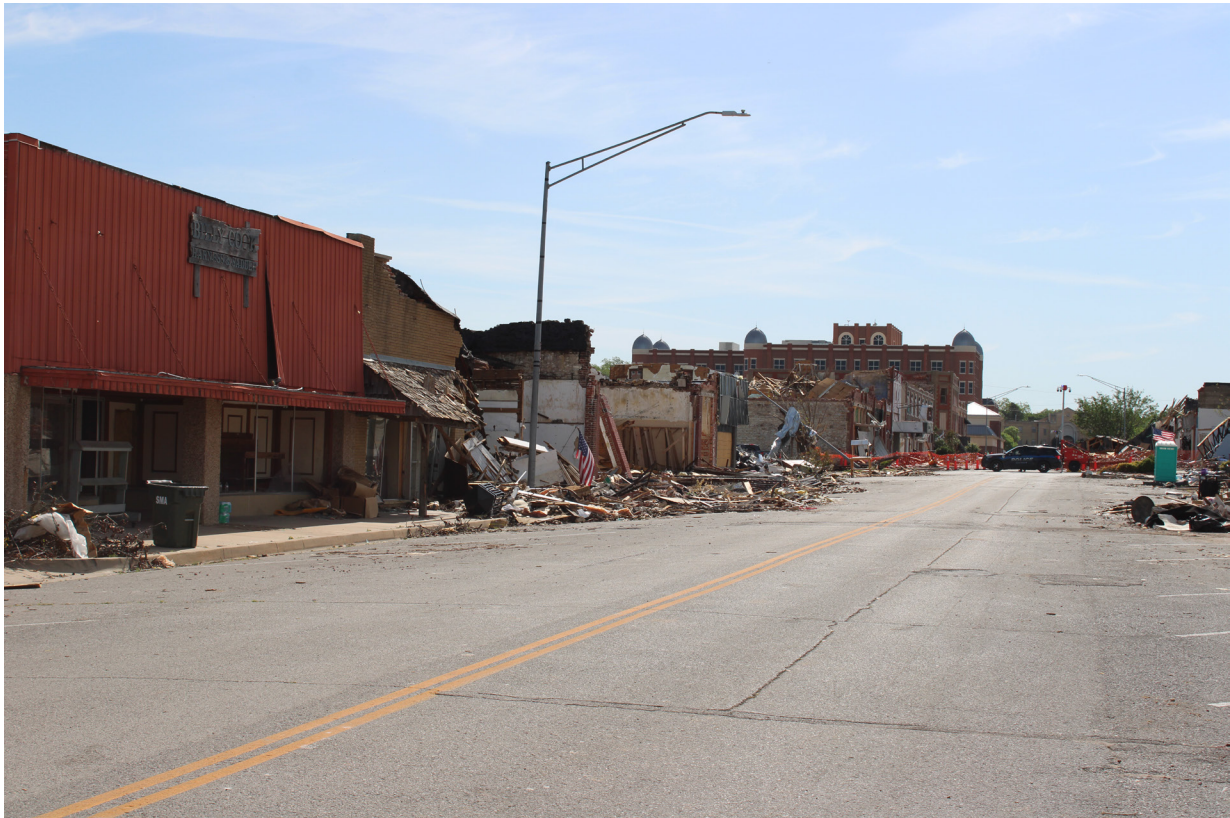
Downtown Sulphur, April 27, 2024, tornado damage
