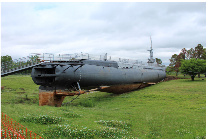
Damage to the USS Batfish from May 2019 flooding, Muskogee, Muskogee County. Photo: FEMA.
