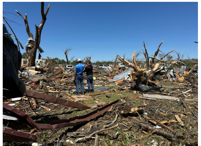
Damage from an EF4 tornado that hit Barnsdall, Osage County, on May 6, 2024. Photo: National Weather Service, Tulsa.
