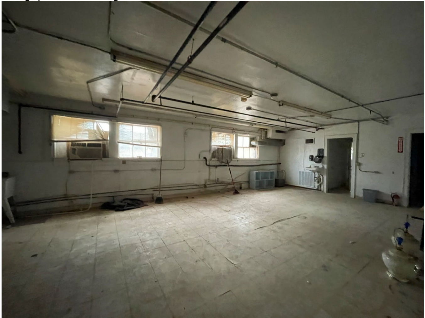
Photograph 9: Interior image of basement level classroom.
