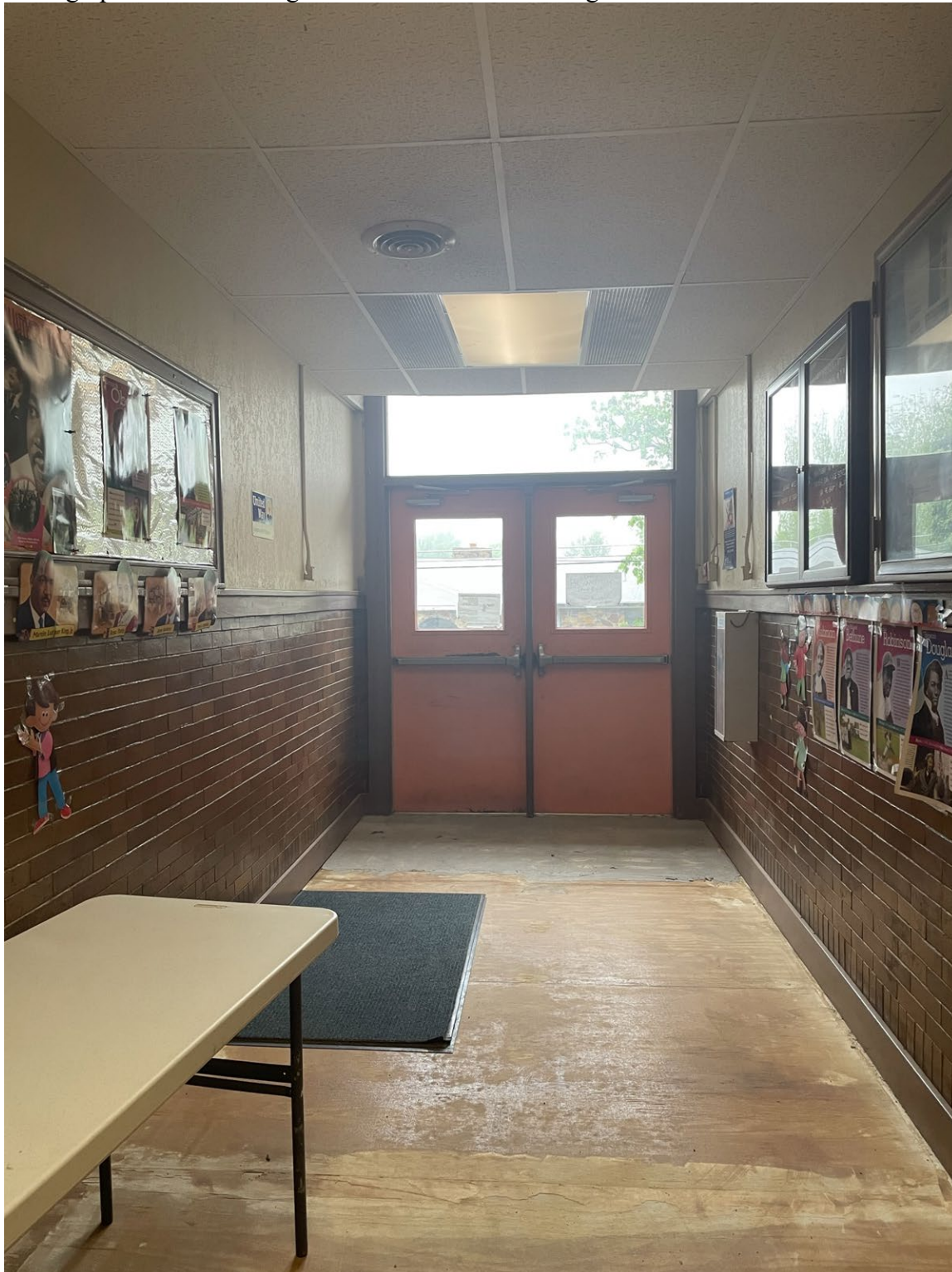
Photograph 5: Interior image of central corridor looking at the main entrance.
