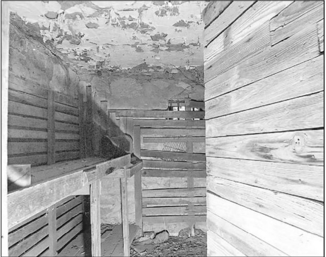
Figure 8. The jail interior in 2002. Source: Daily Oklahoman 2002.
