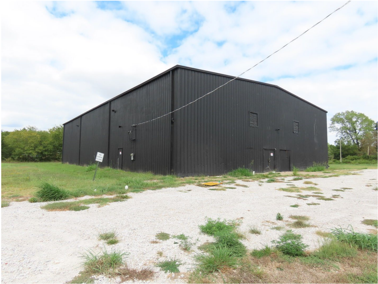
Photograph 32. Oblique of Moton School Gymnasium south façade and west elevation, facing northeast
