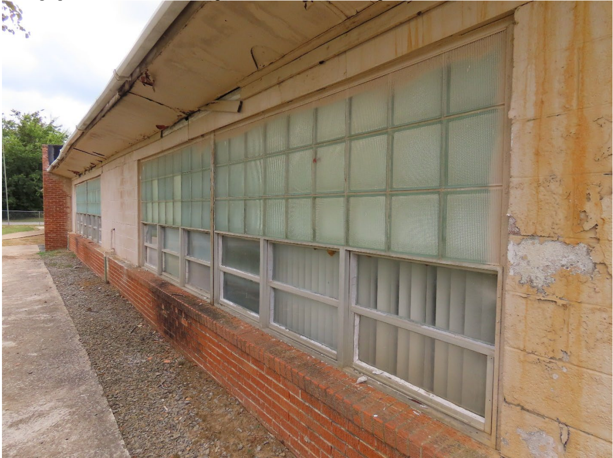
Photograph 8. Detail of Moton High School windows, facing southwest
