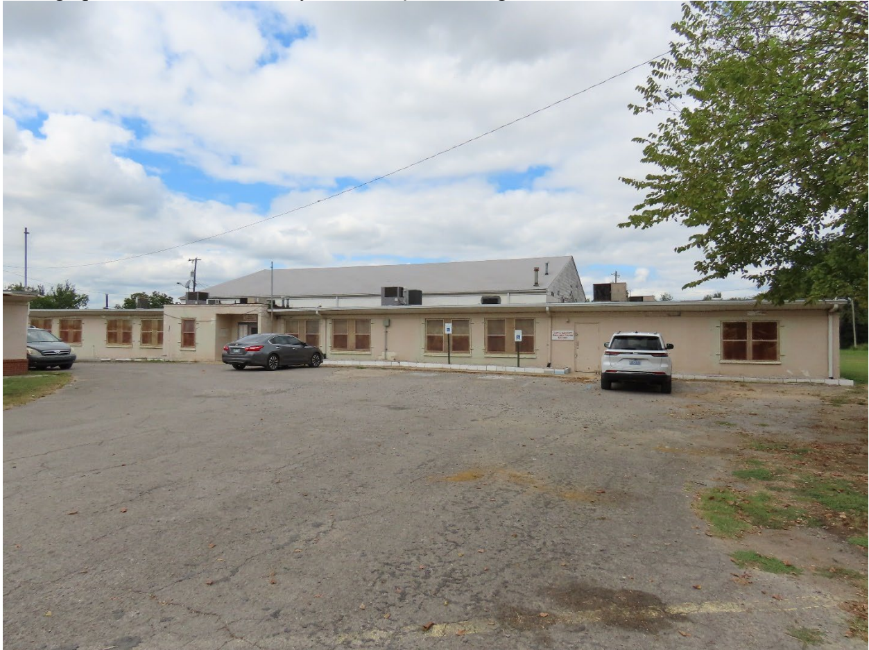
Photograph 19. Moton Elementary School façade, facing northwest
