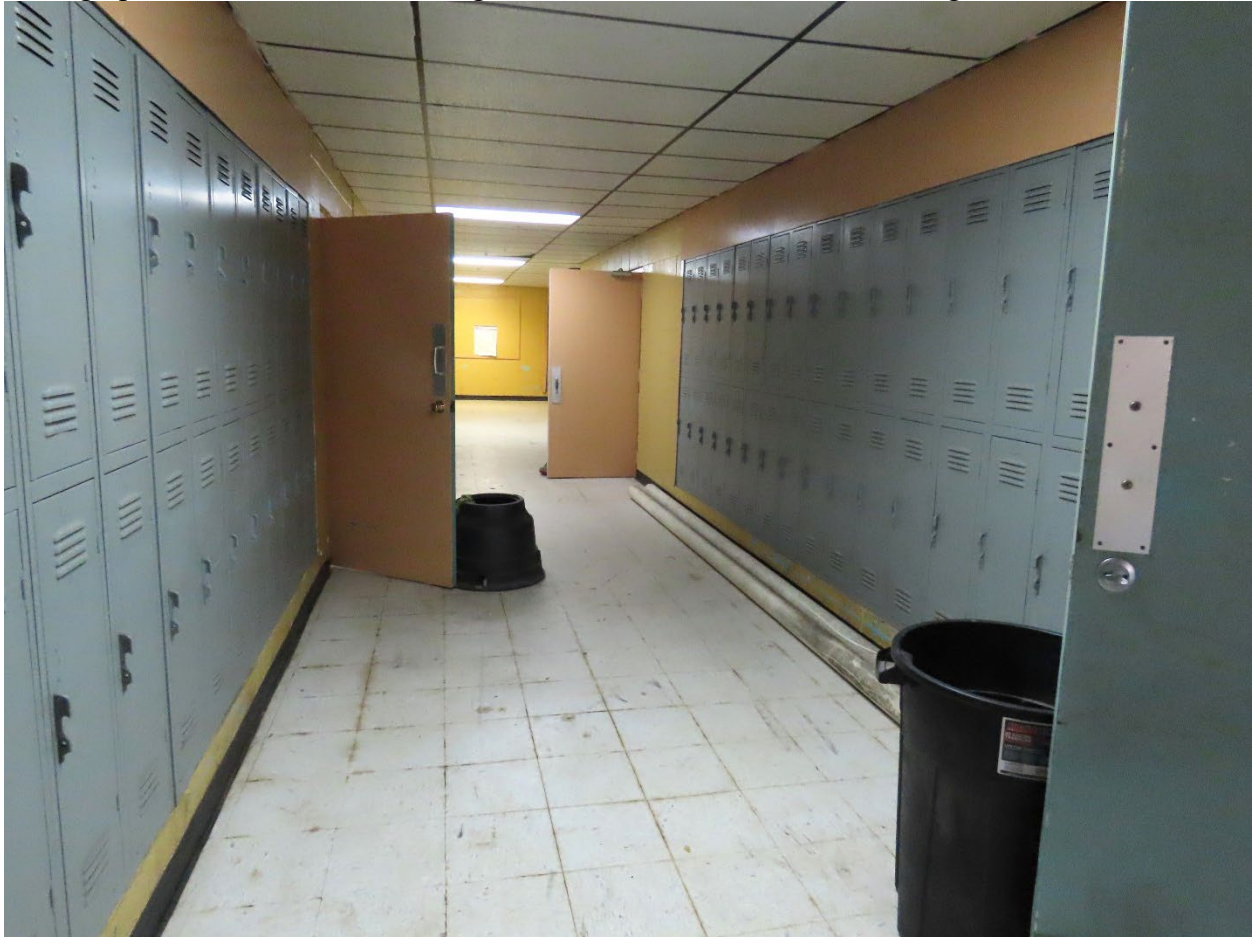
Photograph 13. Interior of Moton High School north-south corridor, facing south
