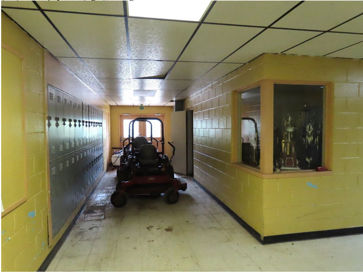
Photograph 12. Interior of Moton High School east-west corridor with bulletin board and lockers (left) and trophy case (right), facing west
