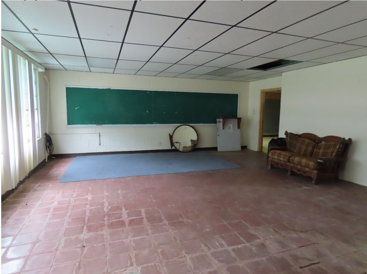
Photograph 14. Interior of Moton High School classroom, facing southwest
