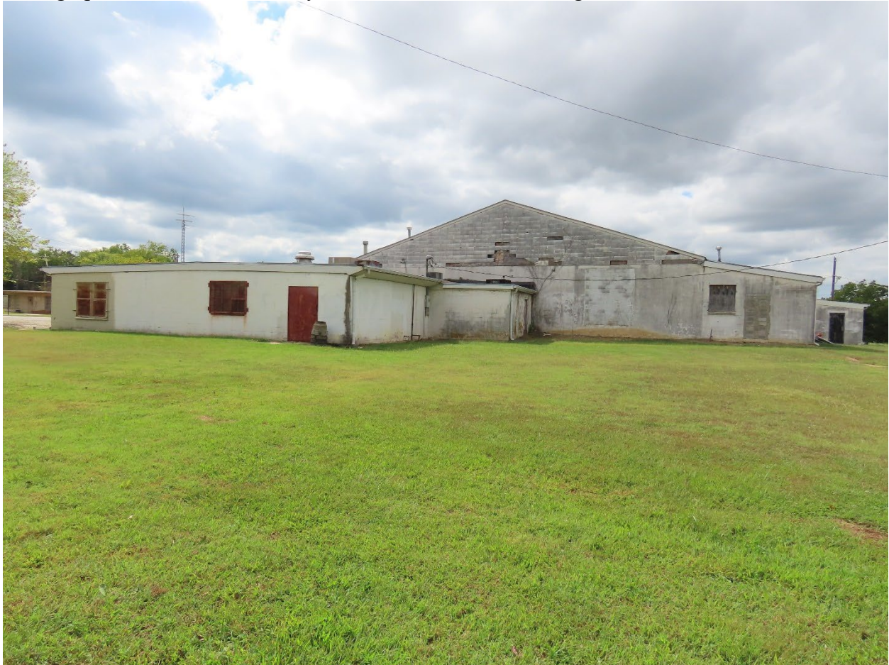
Photograph 22. Moton Elementary School east elevation, facing southwest
