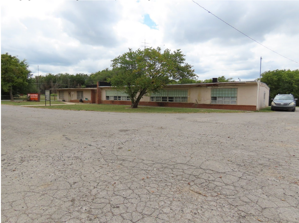
Photograph 5. Moton High School façade, facing southwest
