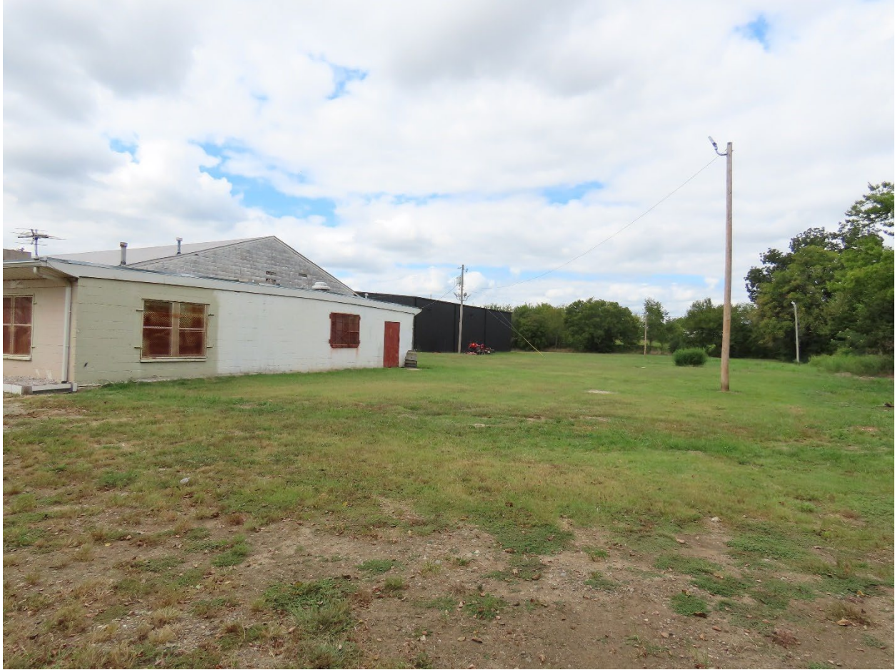
Photograph 3. Overview of Moton School Campus with Moton Elementary School (foreground), Moton School Gymnasium (background), and grassy area with light fixtures, facing northwest
