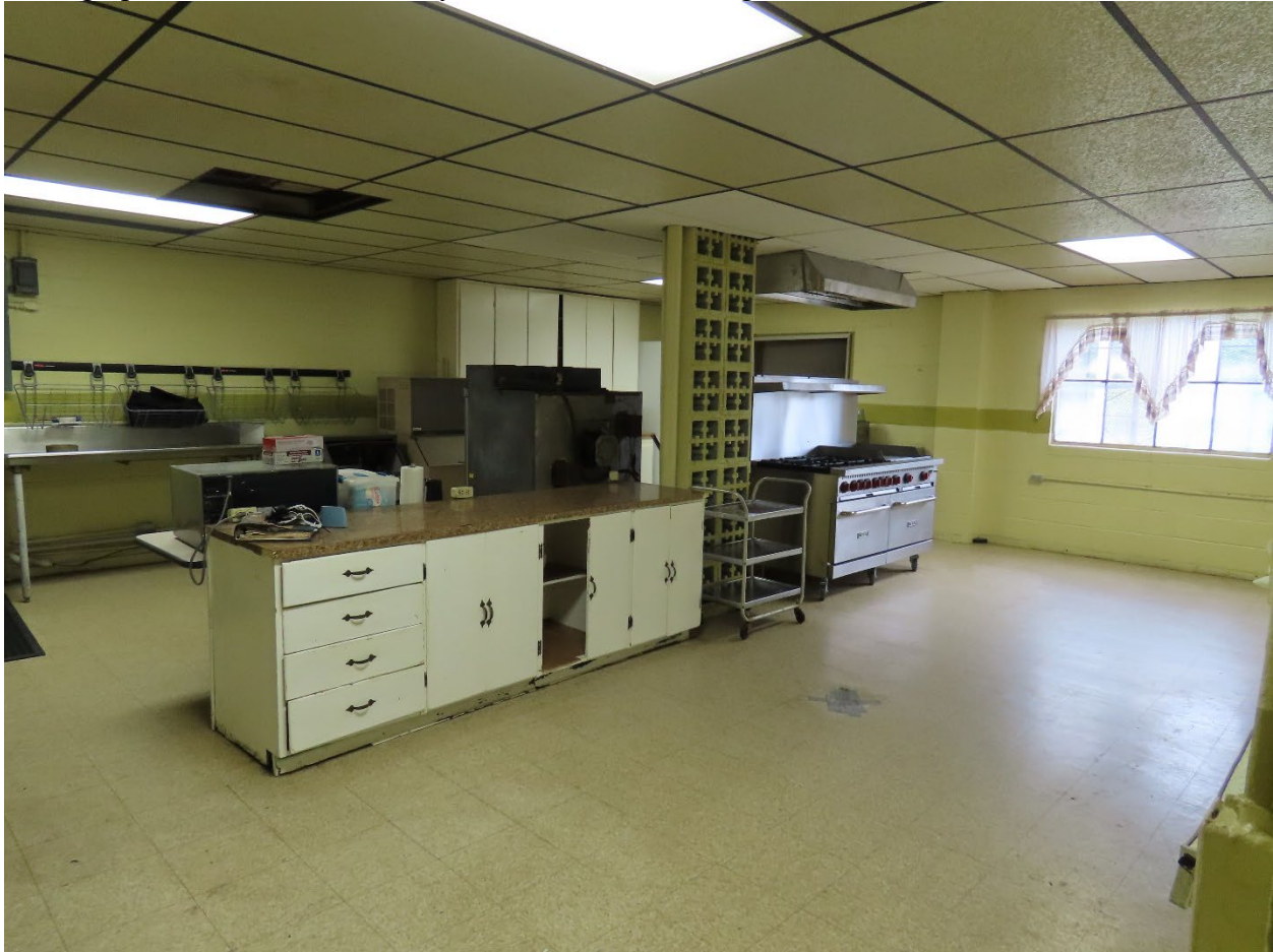
Photograph 29. Moton Elementary School kitchen, facing northeast
