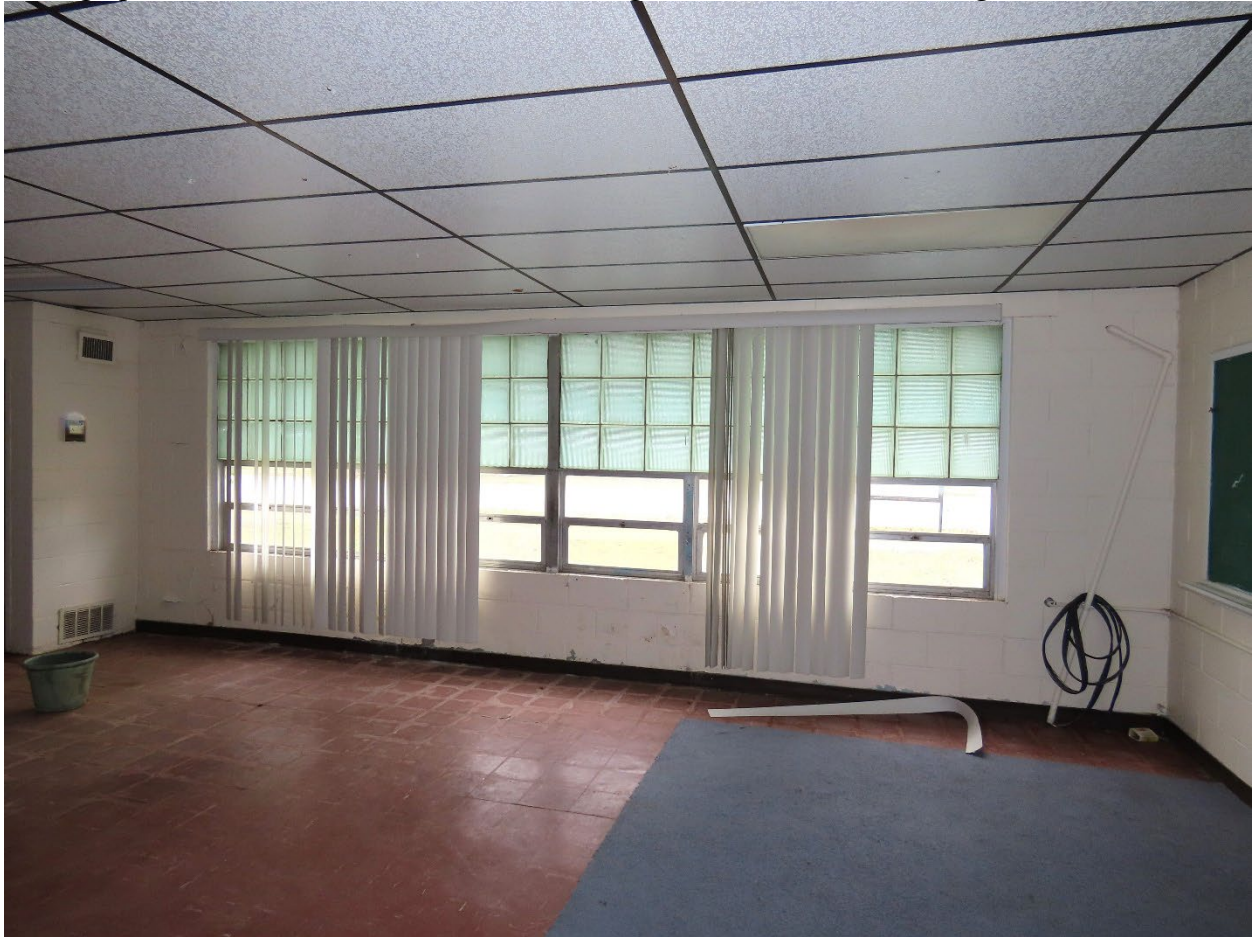
Photograph 16. Interior of windows in Moton High School classroom, facing northeast
