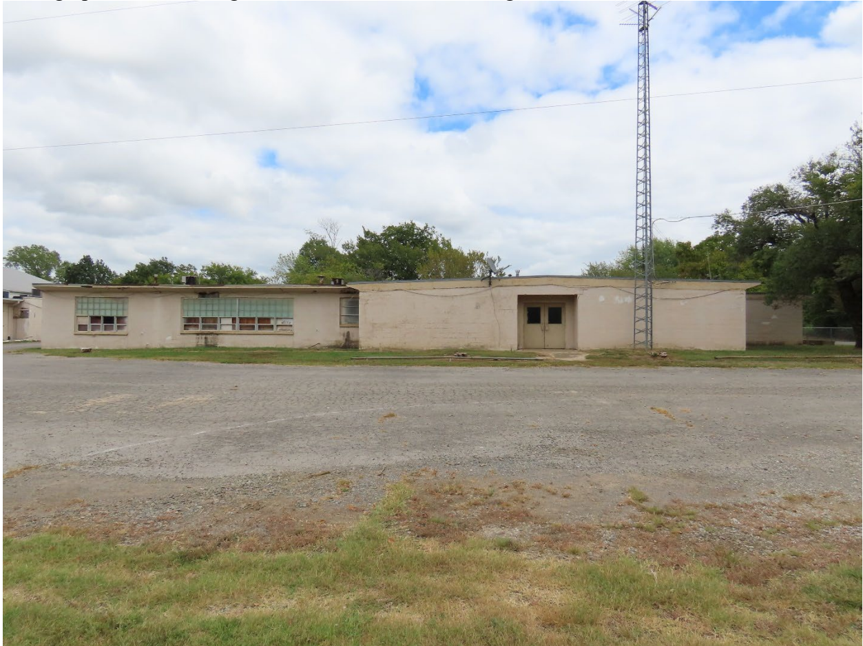
Photograph 10. Moton High School west elevation, facing east
