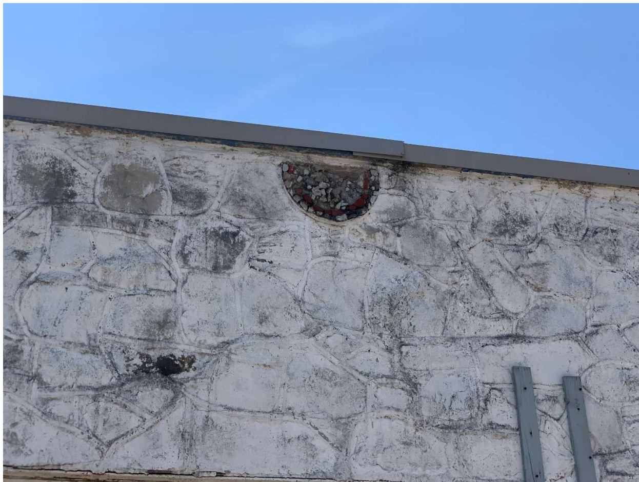
Photo 8: Exterior Facade, Architectural Element, camera facing west.
