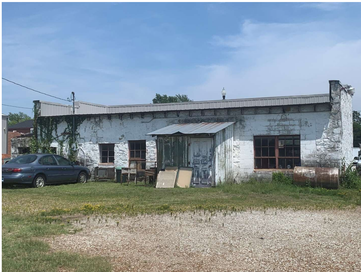
Photo 4: Exterior Facade, camera facing northeast.
