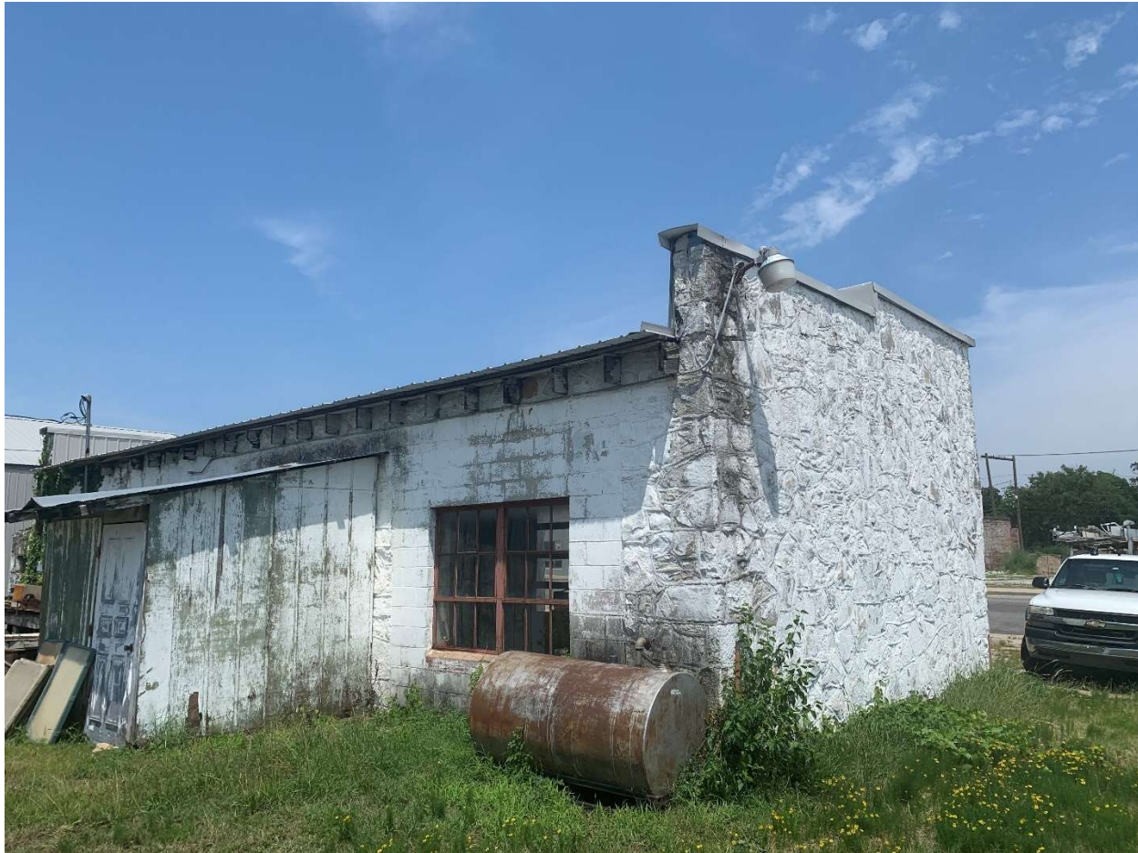
Photo 3: Exterior Facade, camera facing north, northeast.
