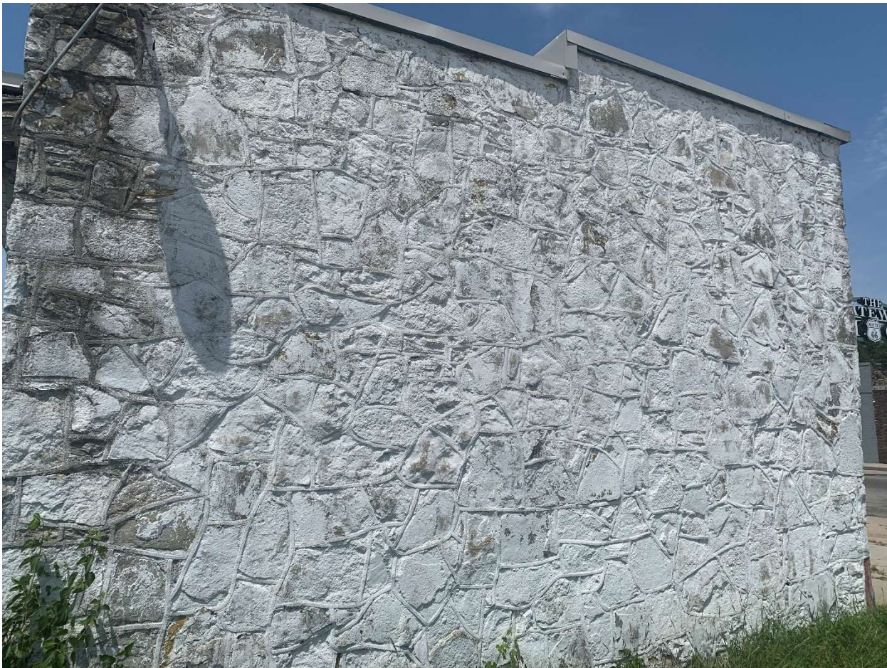
Photo 2: Exterior Facade, focus on existing façade cover, camera facing north.
