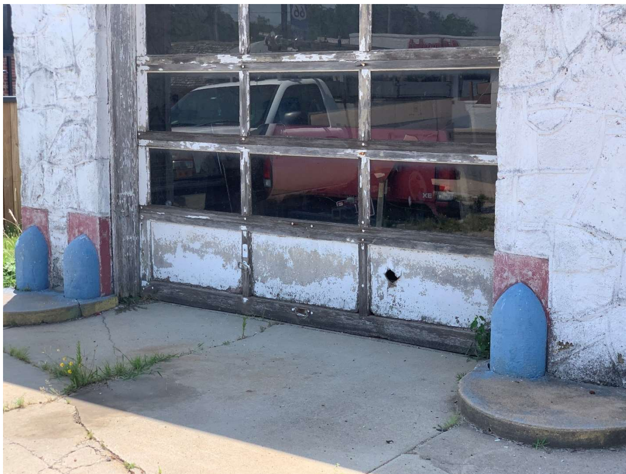
Photo 9: Exterior Facade, Bollards and Garage Door, camera facing west.
