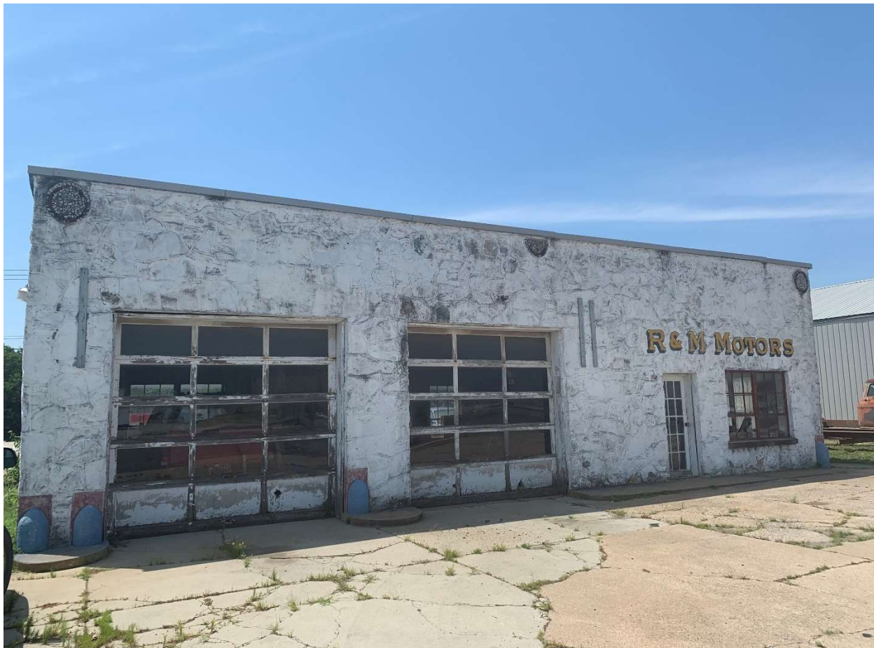
Photo 1: Exterior Facade, camera facing east.
