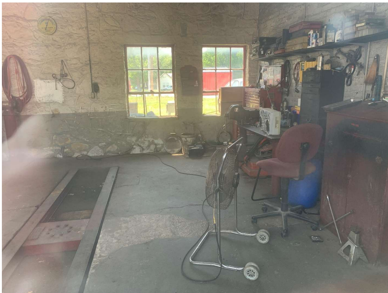
Photo 12: Interior Garage, camera facing west.
