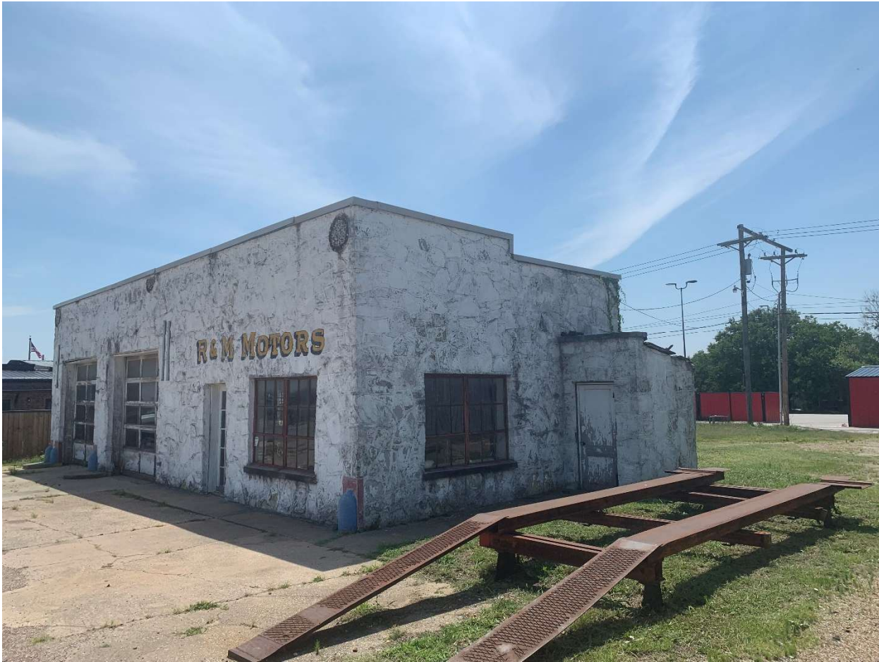
Photo 6: Exterior Facade, camera facing southwest.
