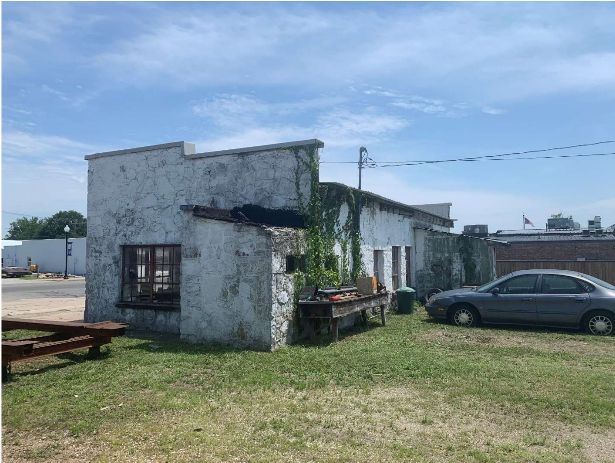
Photo 5: Exterior Facade, camera facing south, southeast.
