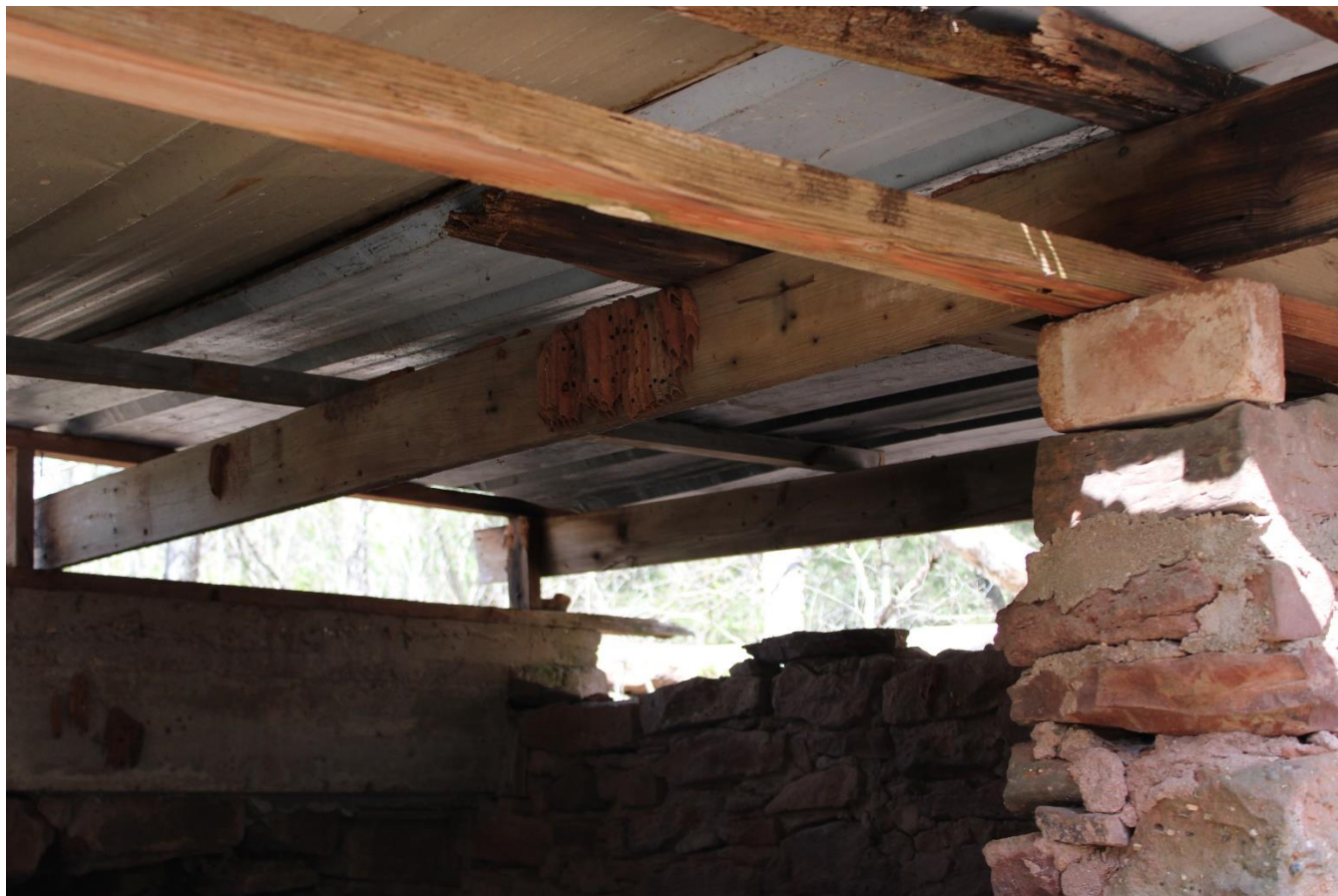
OK_Pottawatomie County_Chisholm Springs Springhouse_0013
