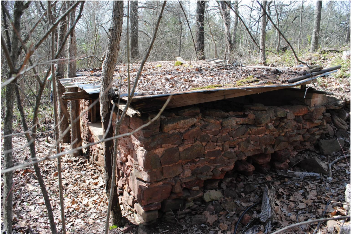
OK_Pottawatomie County_Chisholm Springs Springhouse_0003
