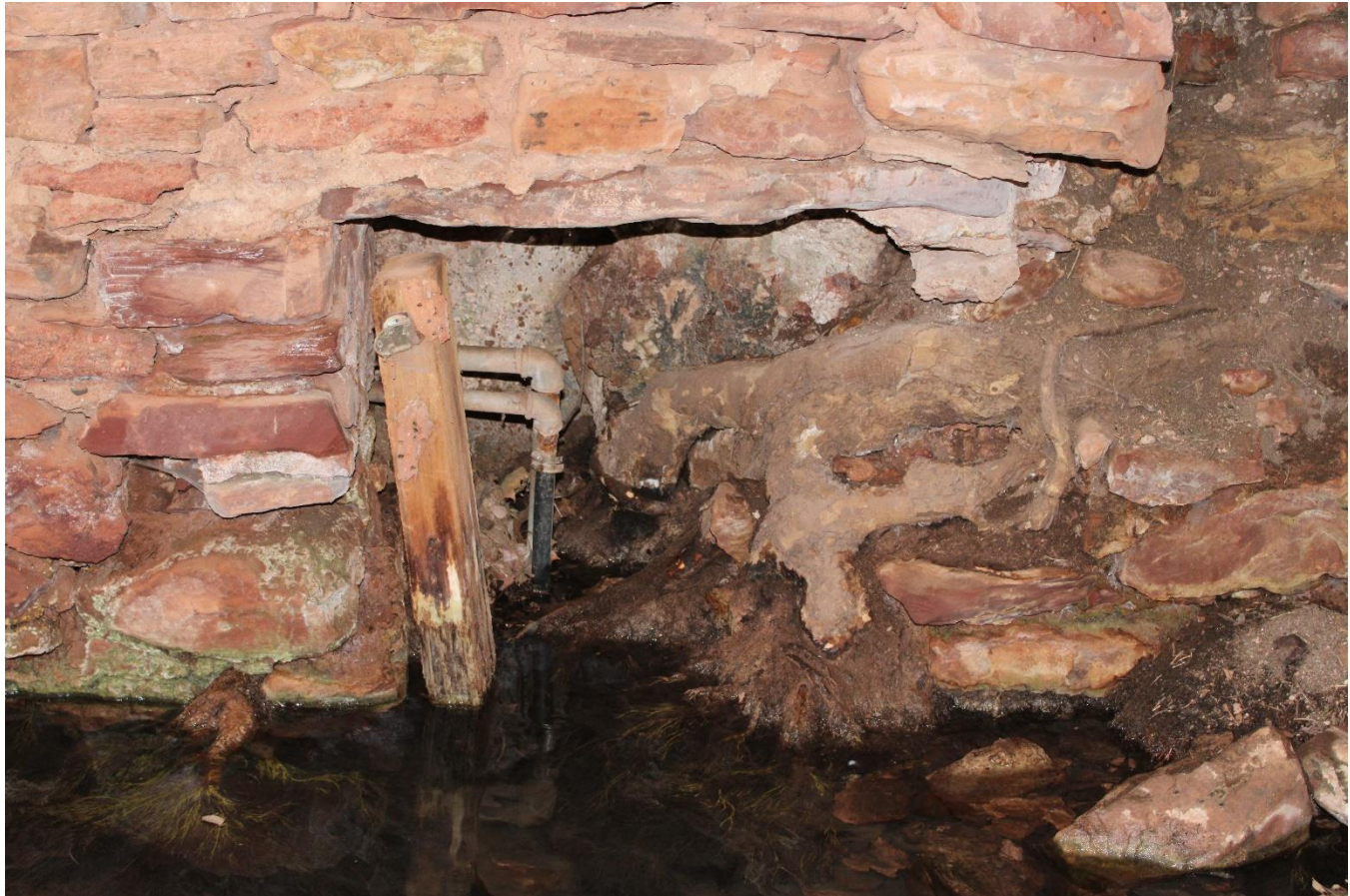
OK_Pottawatomie County_Chisholm Springs Springhouse_0012
