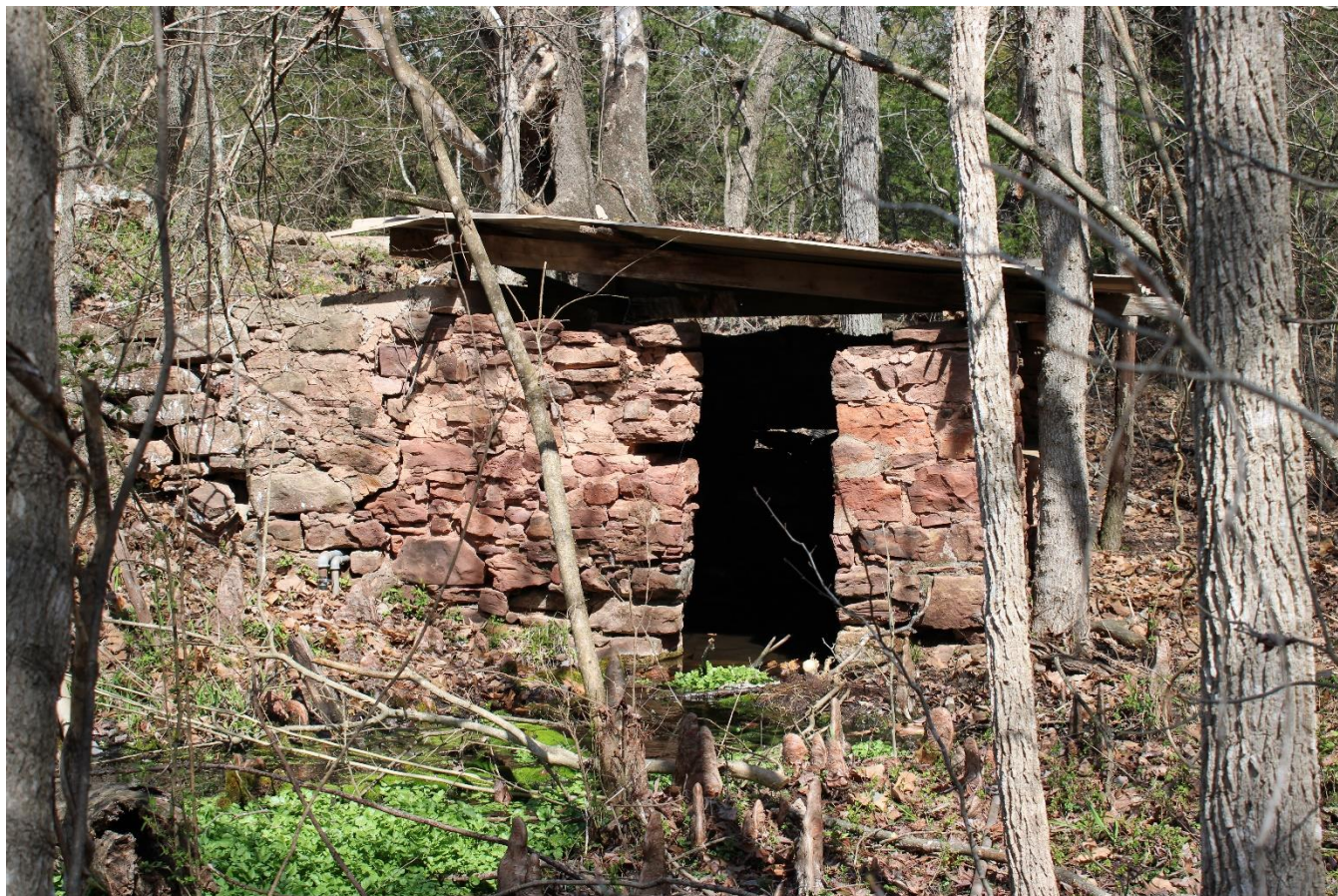
OK_Pottawatomie County_Chisholm Springs Springhouse_0007
