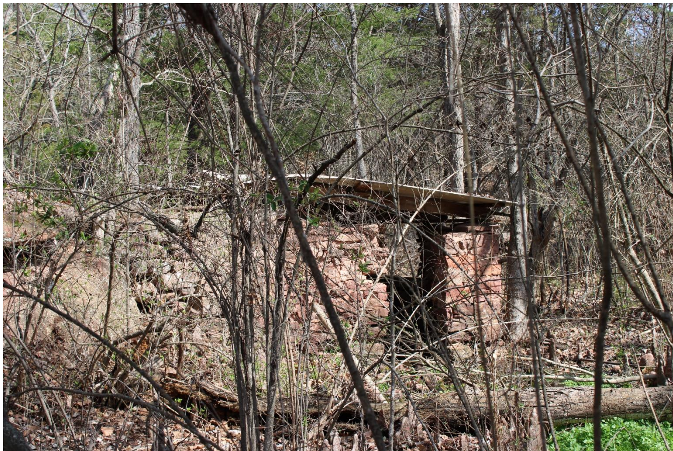
OK_Pottawatomie County_Chisholm Springs Springhouse_0006
