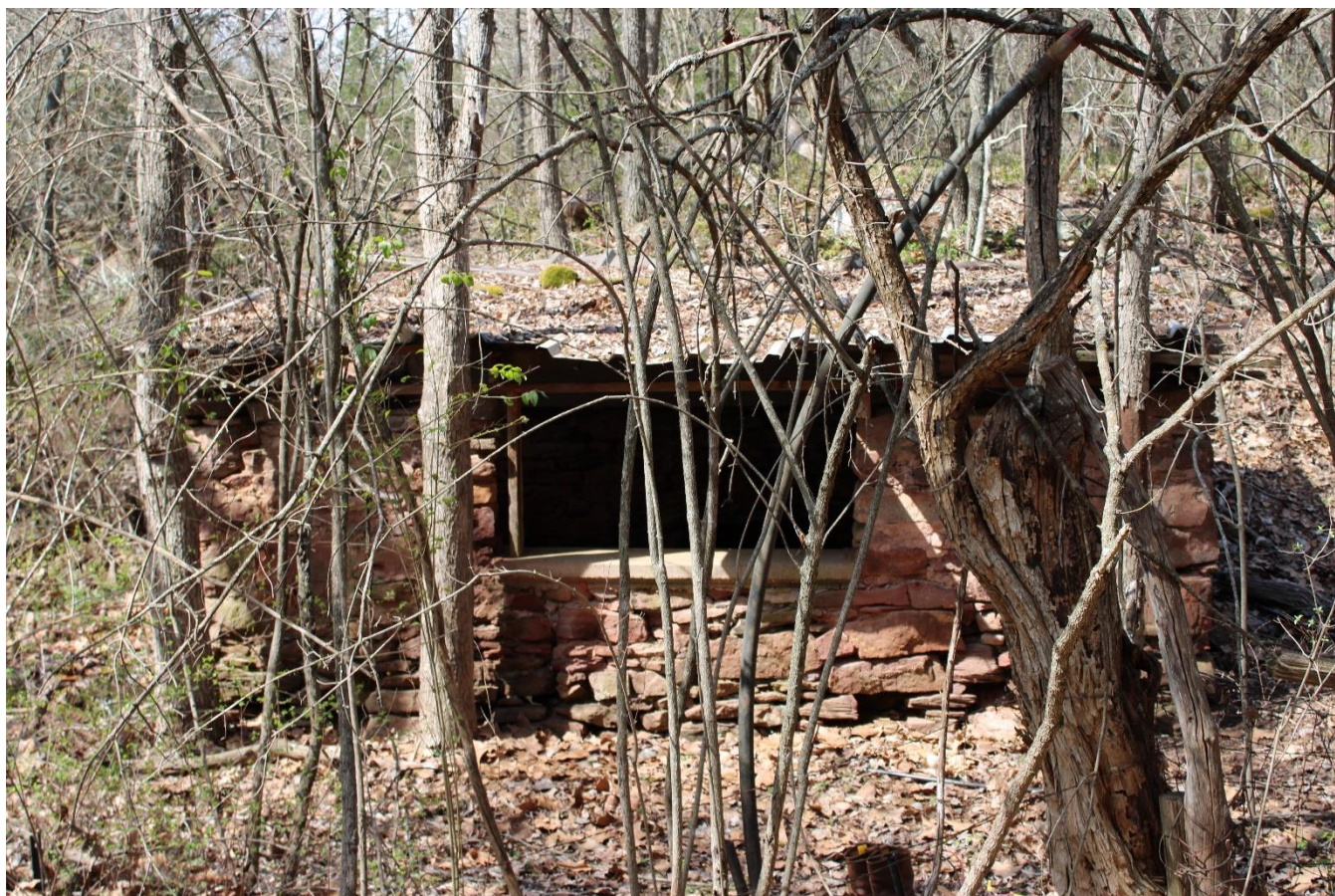
OK_Pottawatomie County_Chisholm Springs Springhouse_0004
