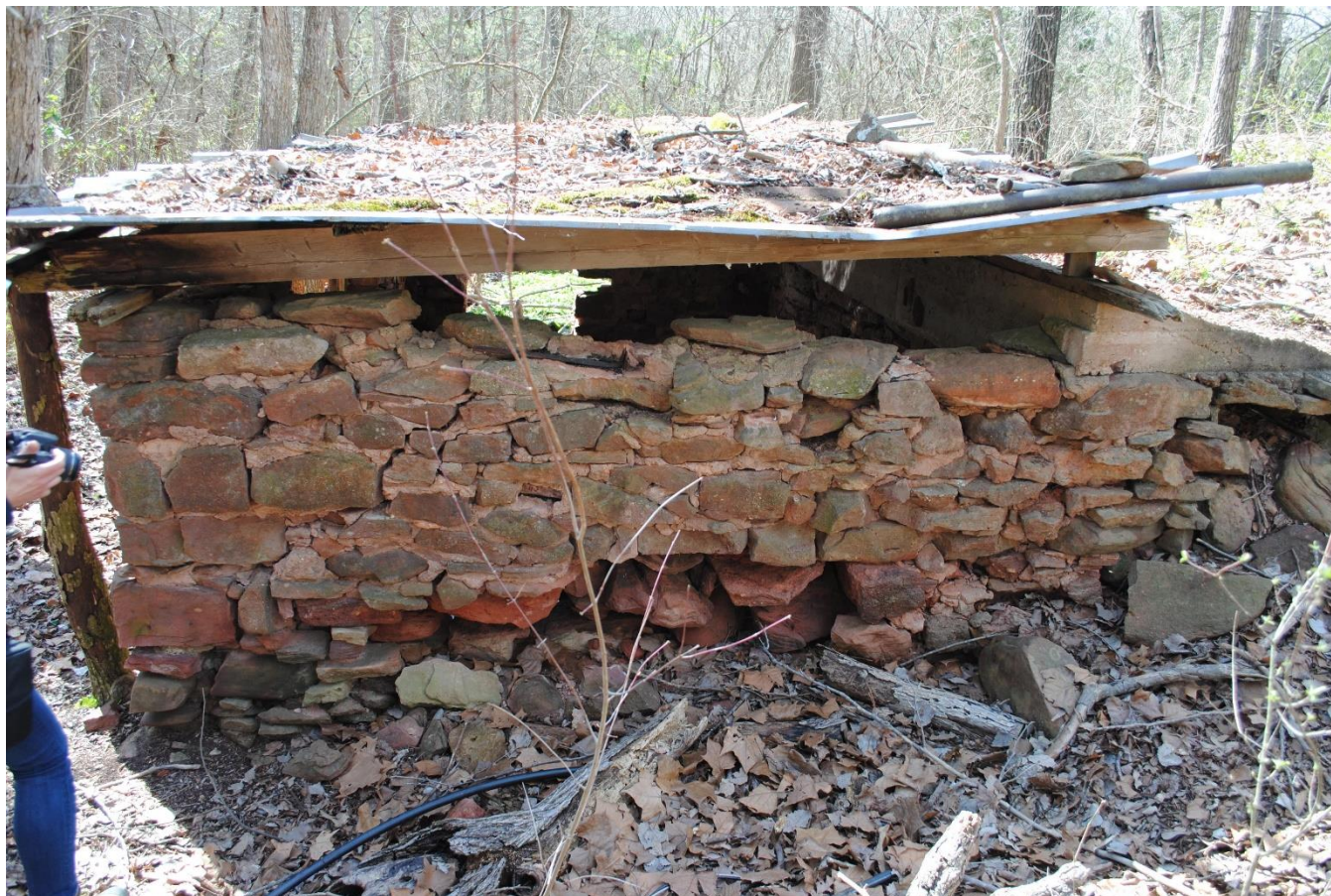
OK_Pottawatomie County_Chisholm Springs Springhouse_0002
