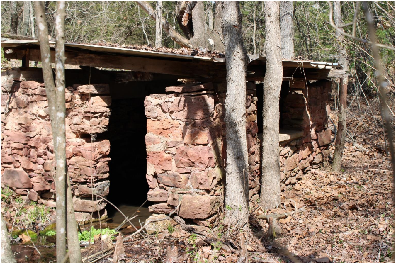
OK_Pottawatomie County_Chisholm Springs Springhouse_0005
