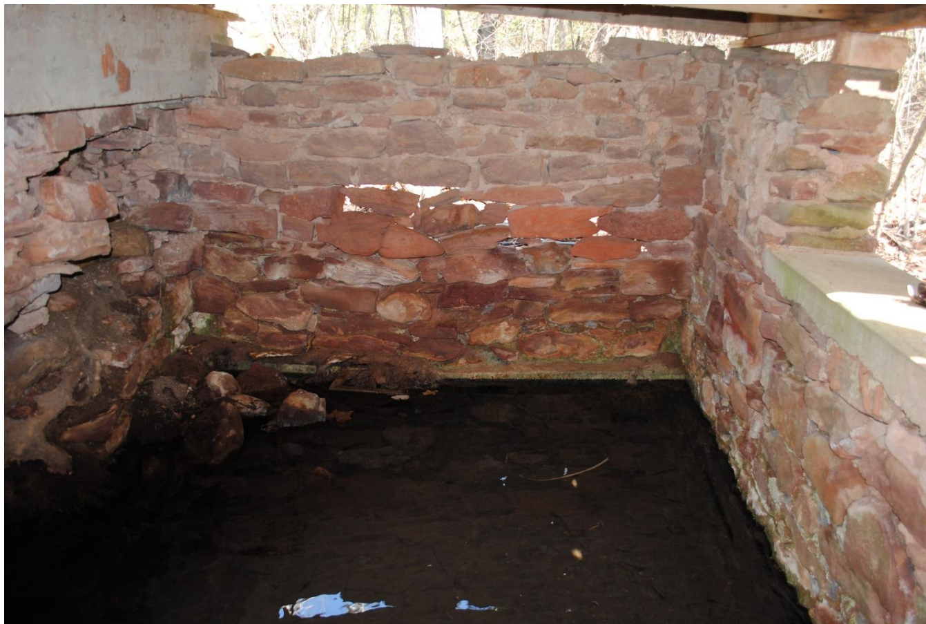
OK_Pottawatomie County_Chisholm Springs Springhouse_0011
