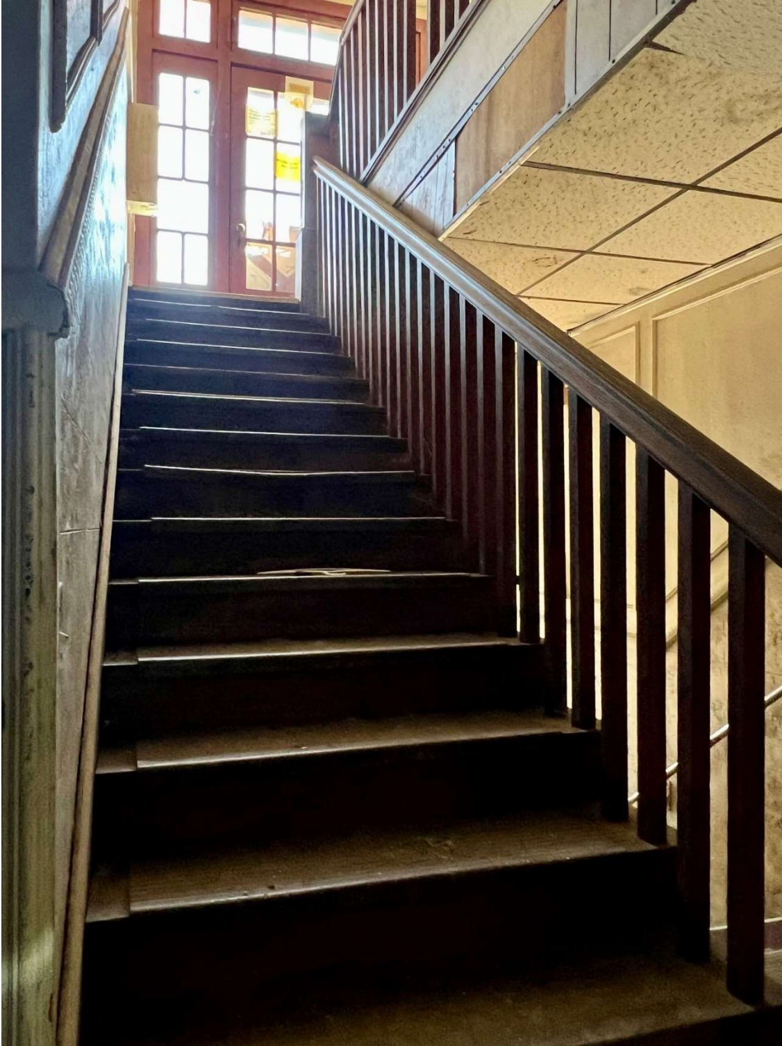
Interior staircase inside the Van-Sanford Apartments. Photo taken looking east.
