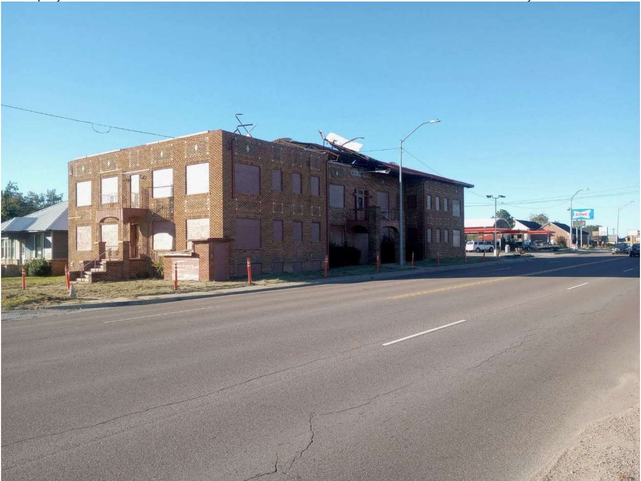
East façade of the Van-Sanford Apartments, front entrance and south façade, secondary entrance. Photo taken facing northwest after the windows were covered.
