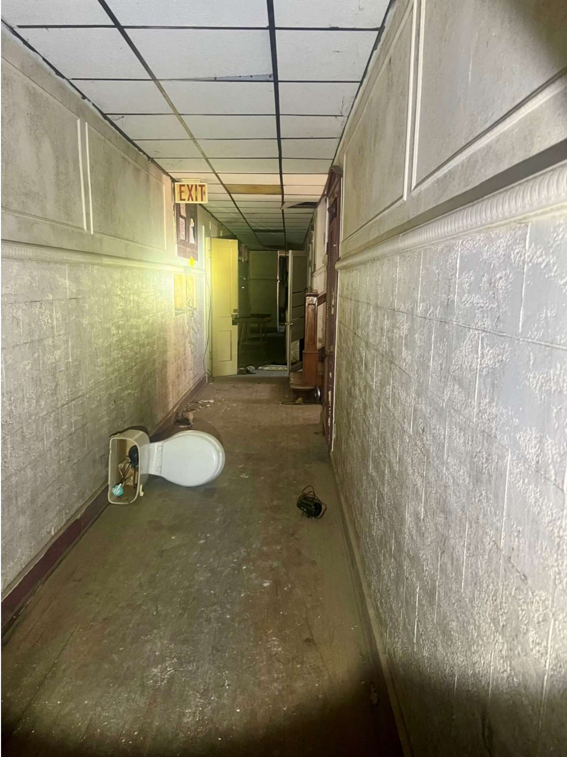
Interior hallway inside the Van-Sanford Apartments. Photo taken looking north.
