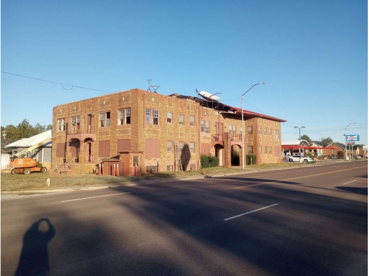
East façade of the Van-Sanford Apartments, front entrance and the south façade, secondary entrance. Photo taken facing northwest before the windows were covered.
