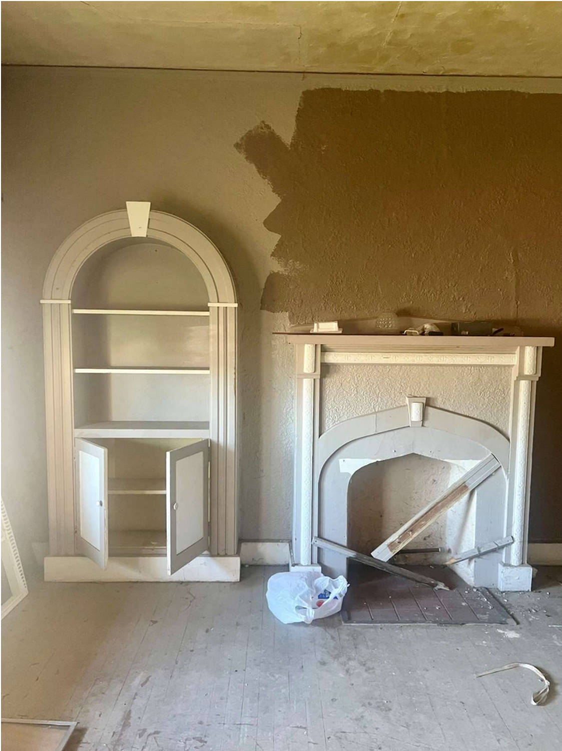
Built-in bookcase and built-in fireplace both with an arch design, in one of the apartments inside the Van-Sanford Apartments. Photo taken looking north.
